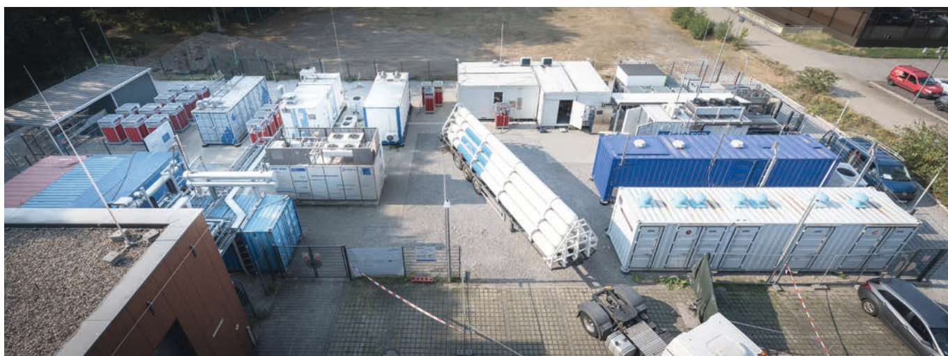
Electrolysis systems and components for hydrogen refuelling stations are trialled at the hydrogen test site at the ZBT.
