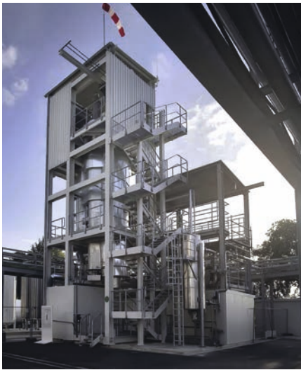
Audi AG's e-gas plant in Werlte provides 1,500 gas-powered vehicles a year with climate-neutral fuel. At the heart of the plant is a methanation reactor from MAN.
