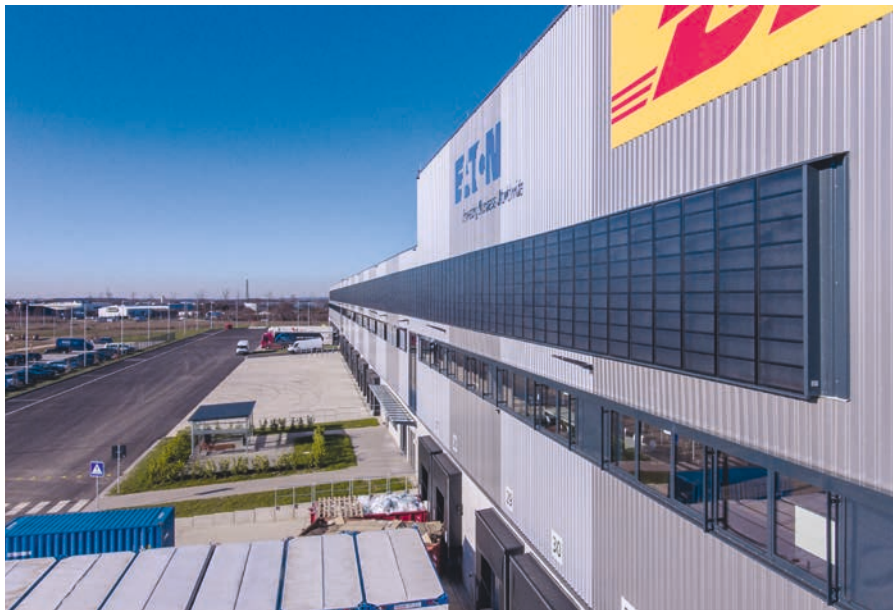
Low-CO 2 building with solar air collector, which efficiently converts solar energy into heat via the medium of air.
