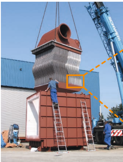
New high-performance recuperator: same level of performance, 25 times smaller in size.
