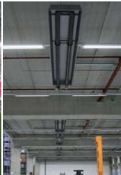
Heating of logistics halls with low-intensity heaters
